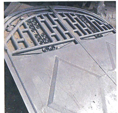
Heavy steel doors placed!
